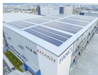
Solar panels at Kansai Logistics Center (installed in June 2021)
