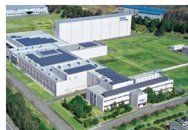
Solar power generation panels at the Shiga Factory
